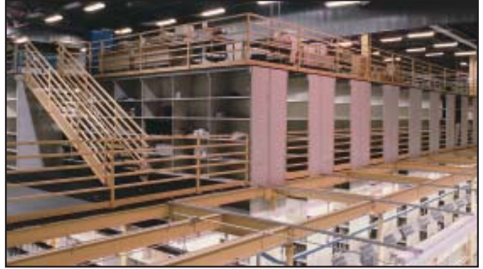
Multi-level shelving with open deck above second level.
